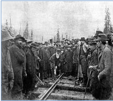
Driving the Last Spike
