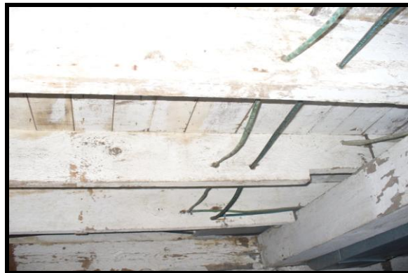
Original beams and support visible in the basement
