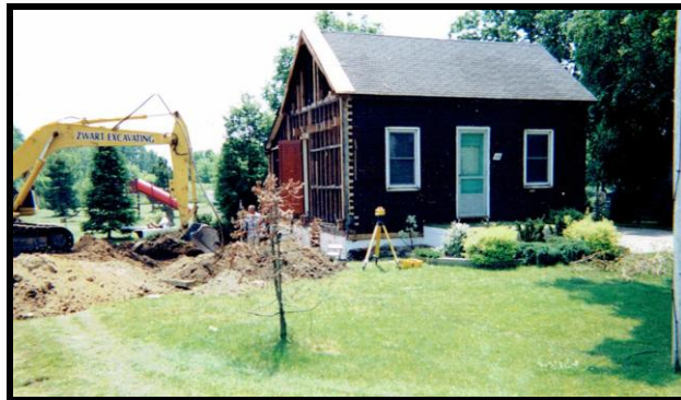
Showing the original building before remodelling
