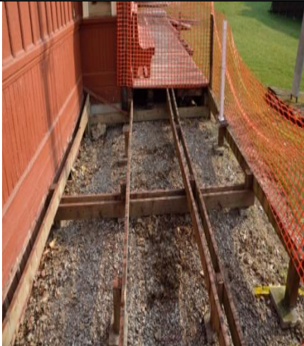
Start of the new section of the deck platform.
